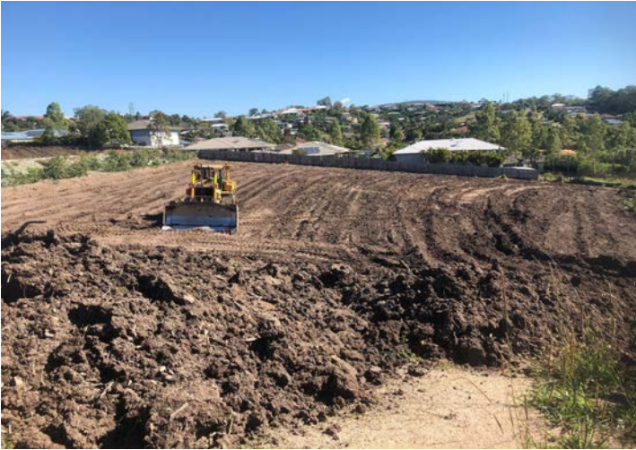
Oversized rock/boulders encountered - removed from area to be filled
