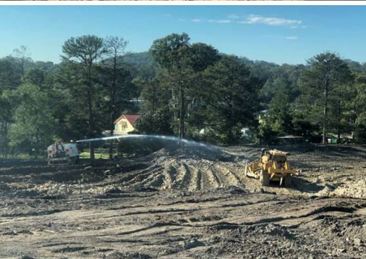
Unsuitable Material - excavated & removed
