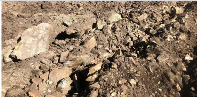
Oversized rock/boulders encountered - removed from area to be filled
