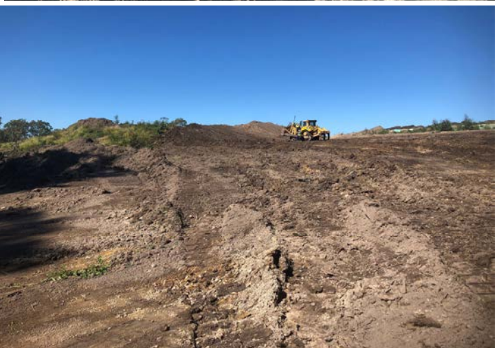
Unsuitable Material - excavated & removed
