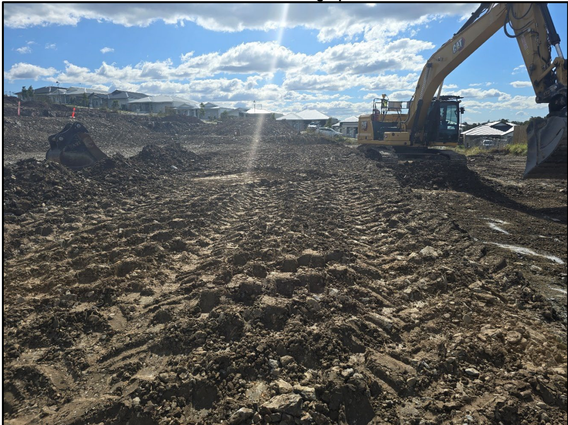
Picture 2: View of Filling Operations
