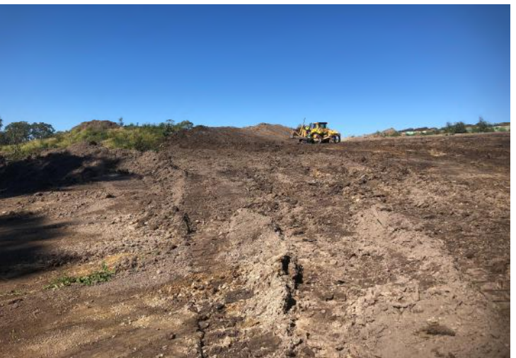
Unsuitable Material - excavated & removed
