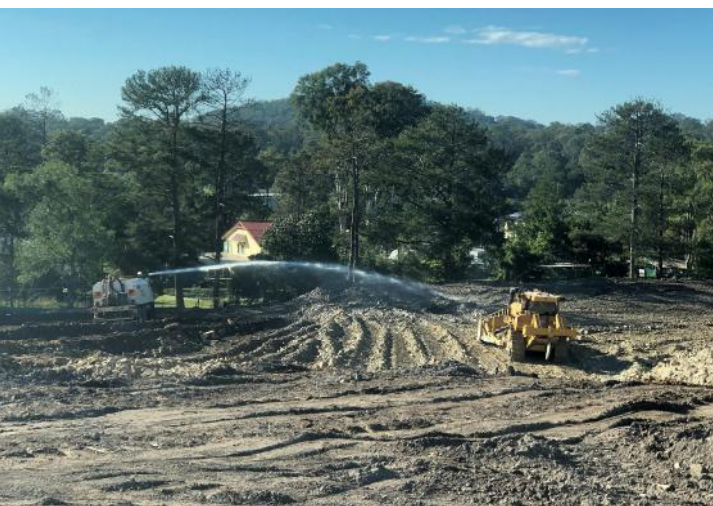
Unsuitable Material - excavated & removed
